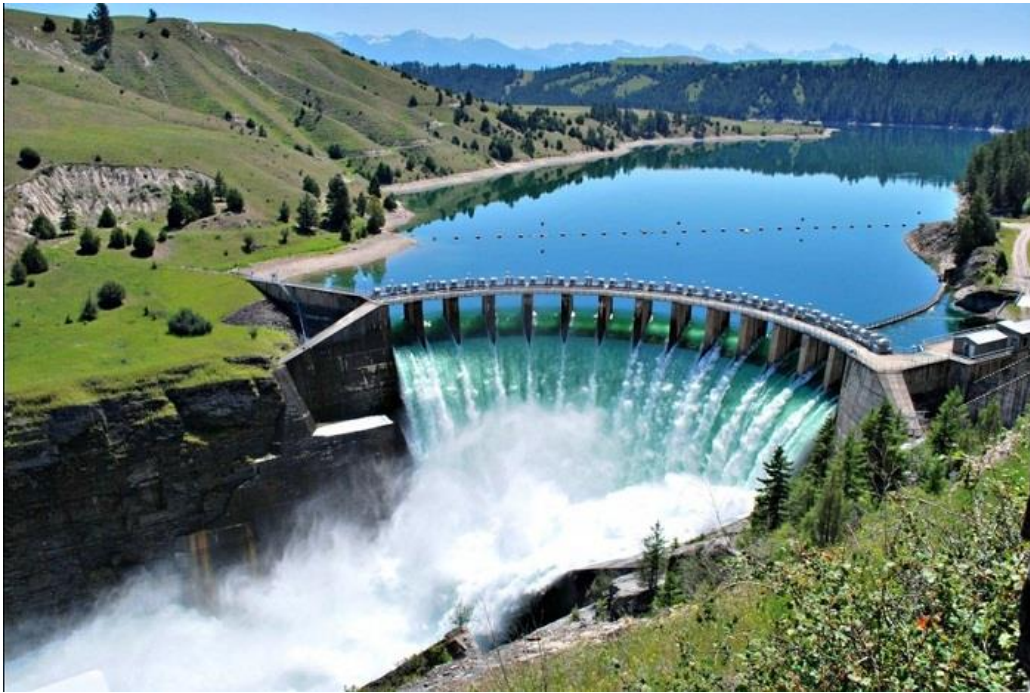
Laúca Hydropower Plant, Angola
